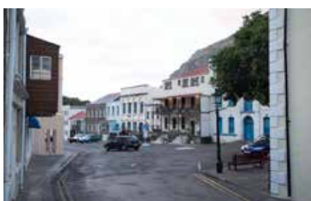
Fig 40. The centre of Jamestown. The site has been proposed as a World Heritage Site due to its British Georgian architecture.
